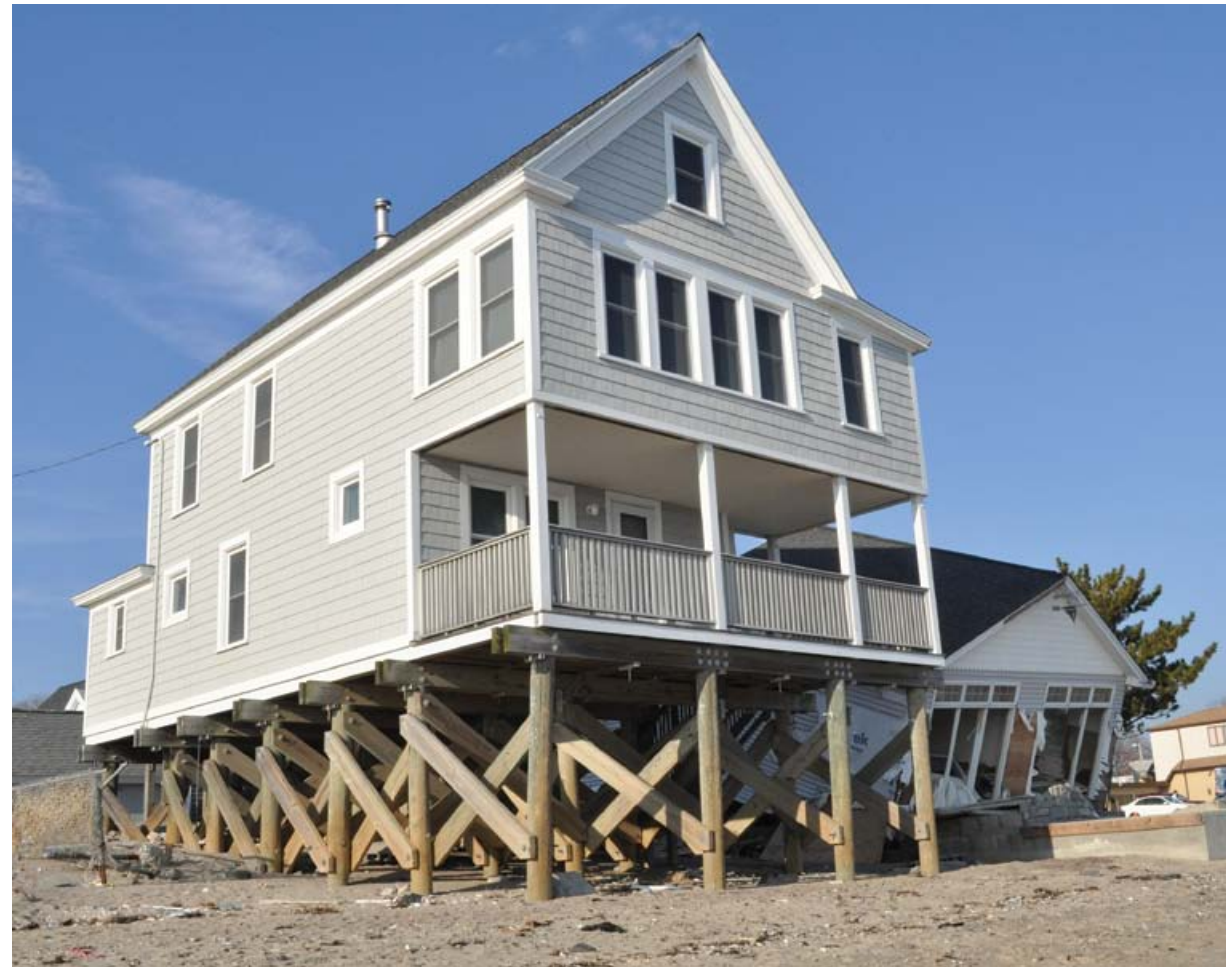
Example of a building on pilings.
