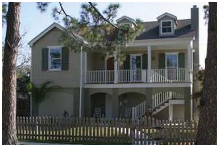
Before-and-after views of whole house elevation, with pier-and-beam construction.
