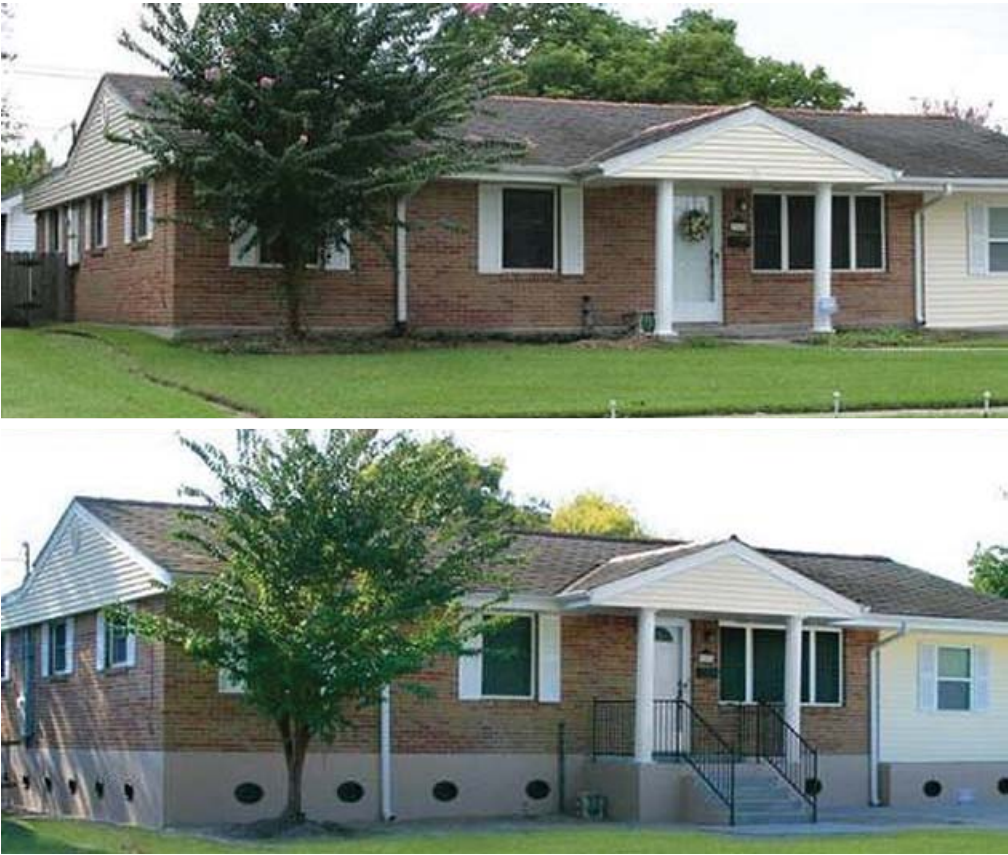
Slab elevation, before-and-after views.
