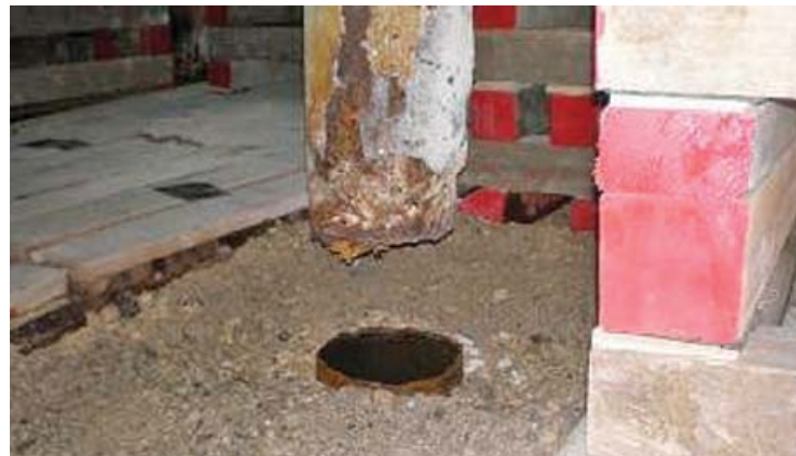
Disconnection of pipe.
