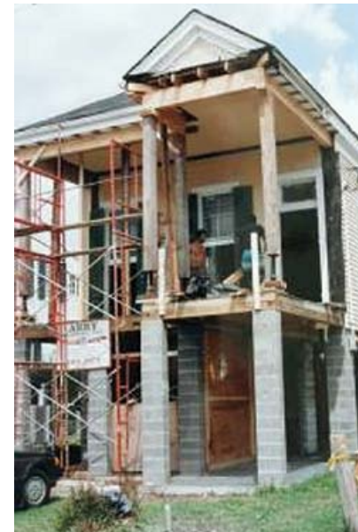
RIGHT: Samuels-Epstein house, during renovation and elevation.
